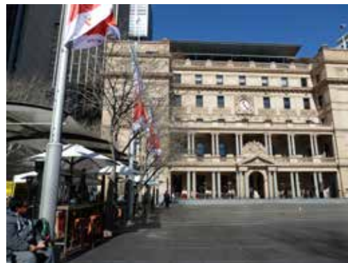
Customs House Square - existing configuration
