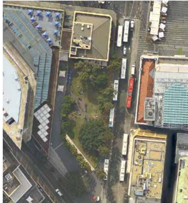
Jessie Street Gardens - aerial
